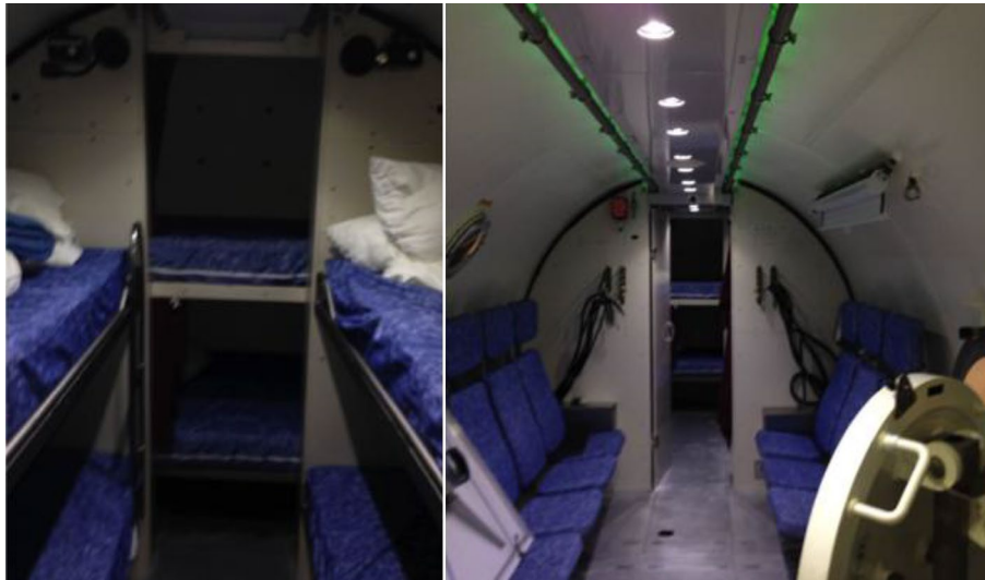
Fig. 1 Image on the left shows the sleeping quarters, shared between 6 divers. The image on the right shows the full length of the living quarters shared by saturation divers for up to 28 consecutive days
